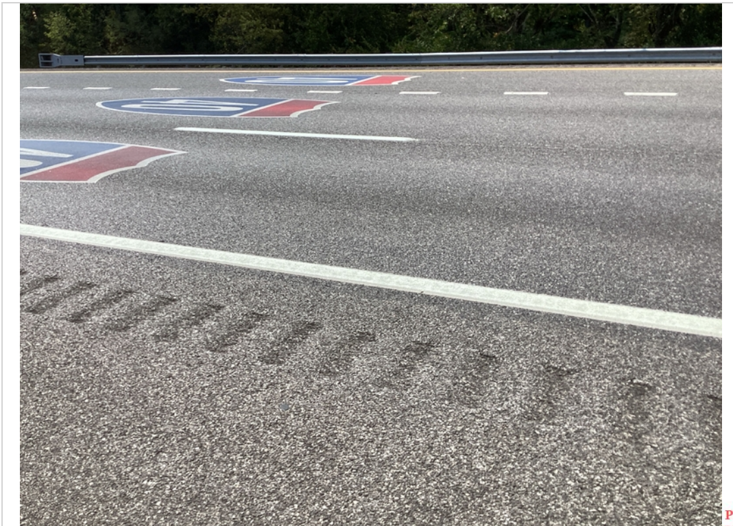
View across culvert wearing surface - northbound lanes
