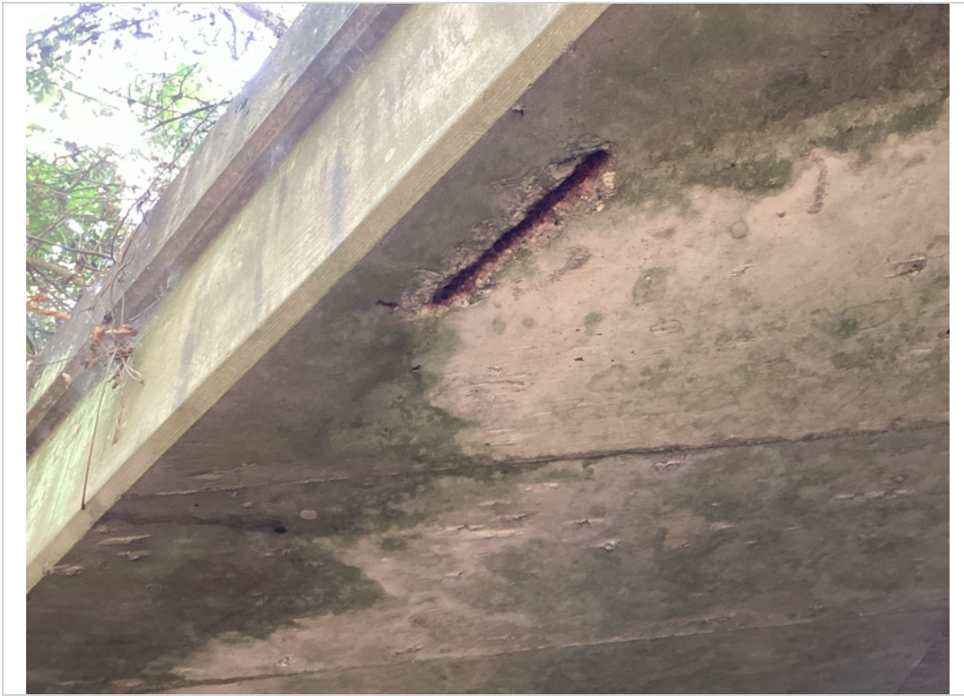
Barrel 1 - Popout top at inlet
