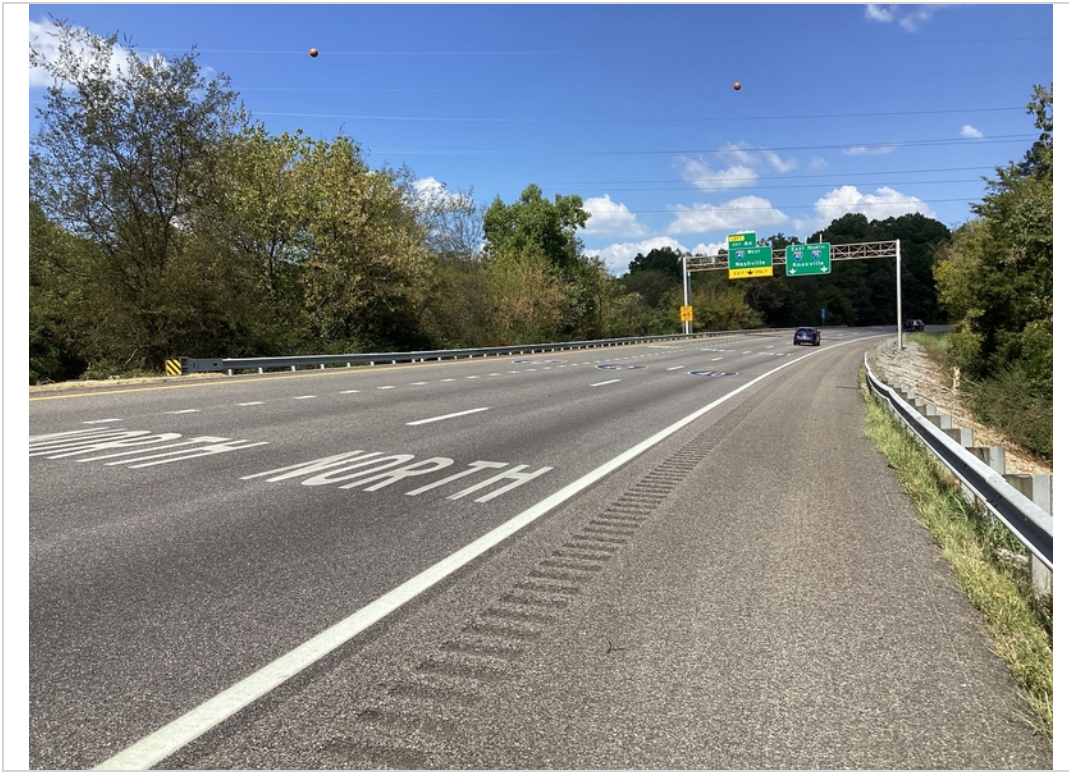
Approach on log - northbound lanes
